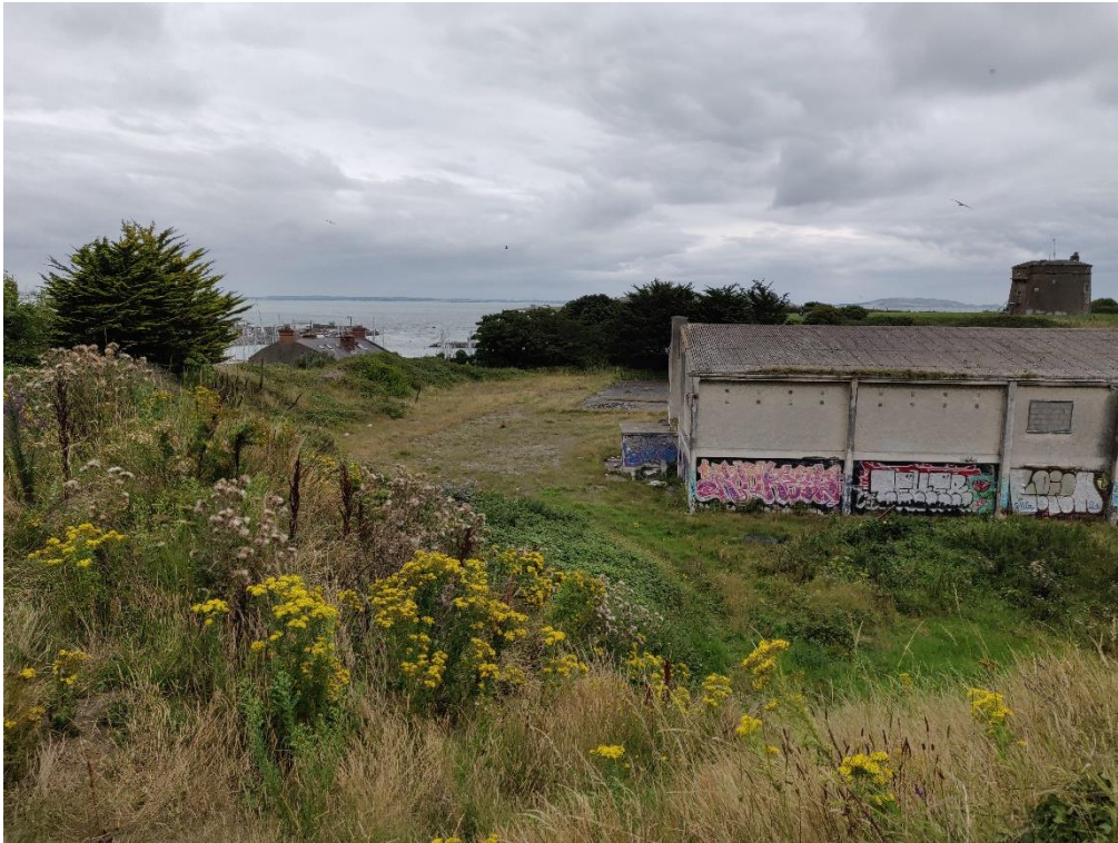
Figure 5-7: Former "Edros Centre", scrub and recolonising bare ground (centre background) at the Site of the Proposed Development. Image taken 16 th August 2021
