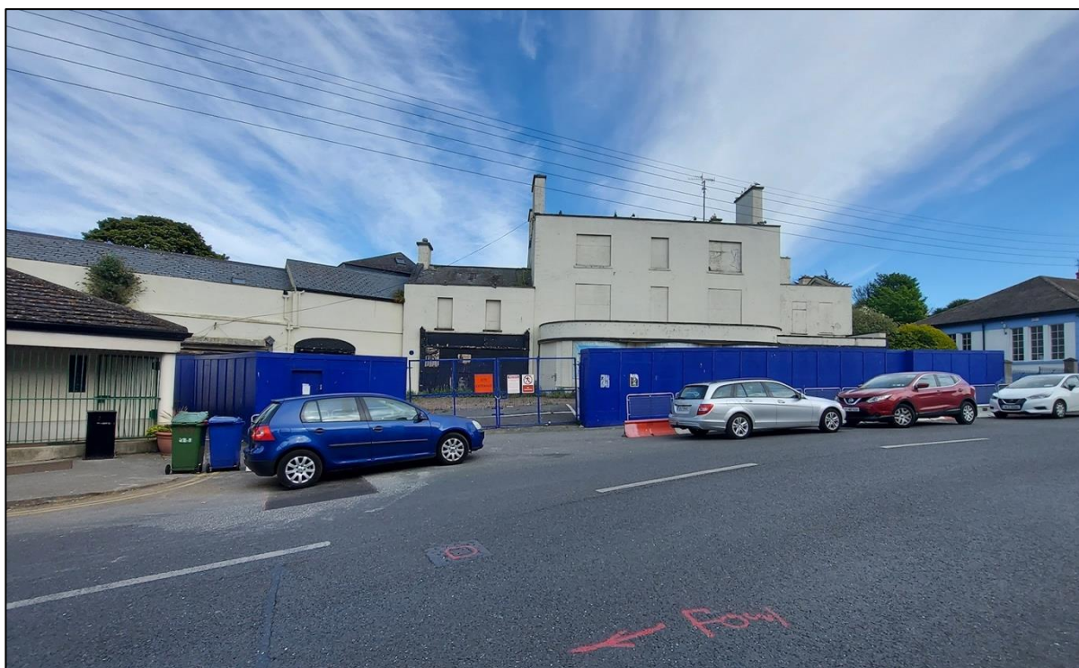
Figure 10-5: The derelict Baily Court Hotel, which aligns the southwest of the site where it fronts onto Main Street in Howth village centre.
