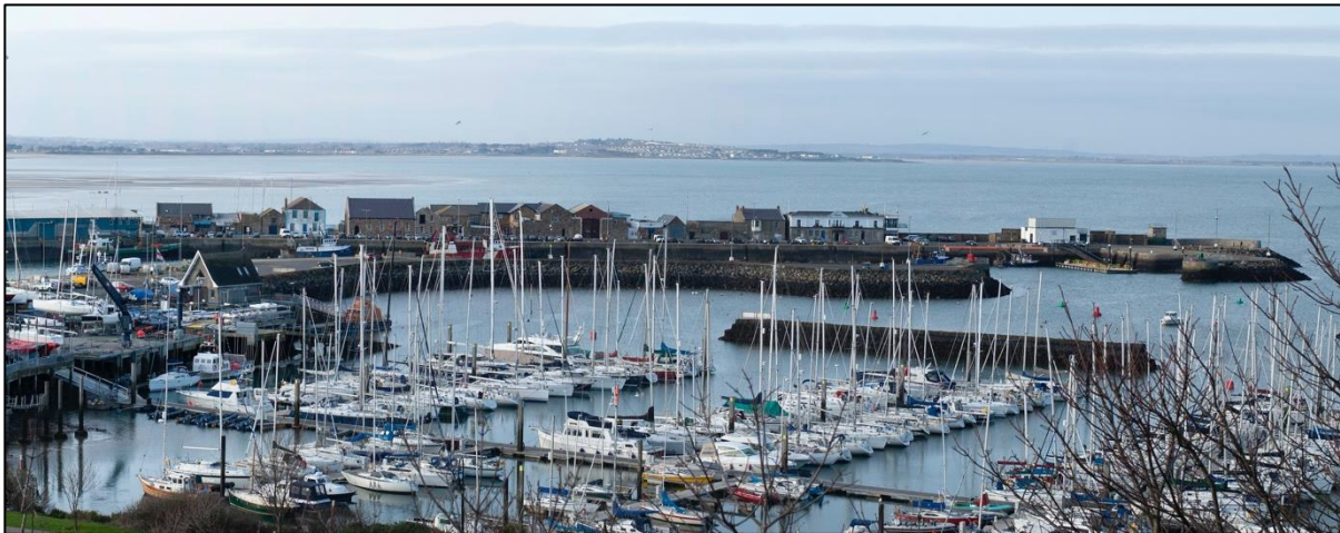
Figure 10-9: View of Howth Harbour from the Martello Tower
