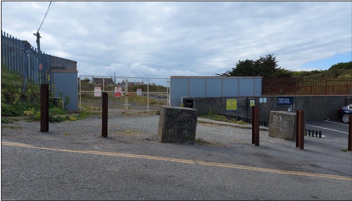
Figure 10-6: The northeast boundary of the site, where it aligns Balscadden Road
