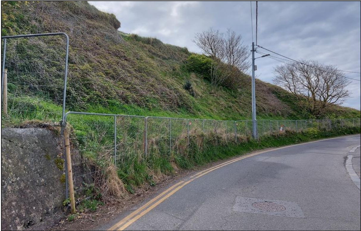
Figure 10-8: Balscadden Road, near the southeast corner of the site
